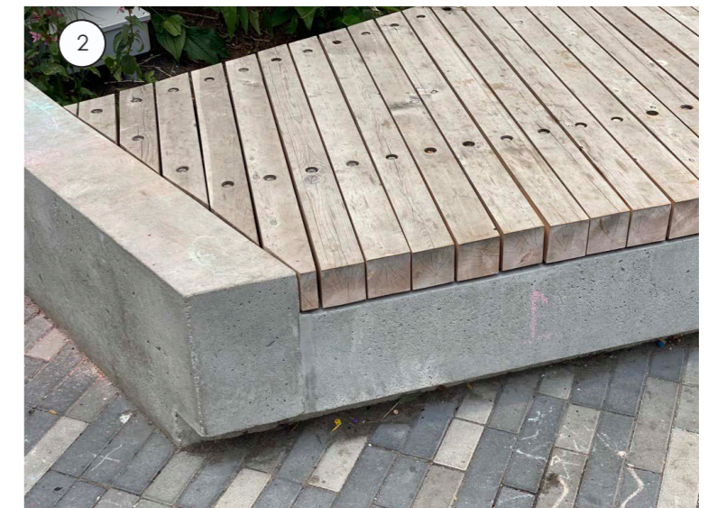
Wide benches of polished concrete, with inset for strip lighting
