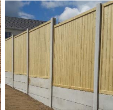
Garden dividers: 2000mm high of proprietary precast concrete post and plank construction, with timber panels above 1000mm. - to arch
