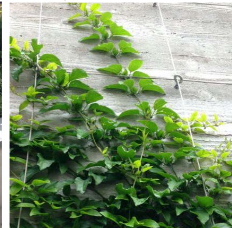
Climbing plants & tension wire against walls in carpark - refer to planting plan
